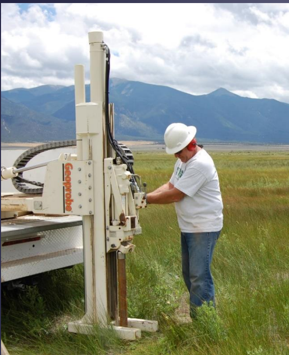
Photograph of Hydrologic Technician Fred Gebhardt installing a piezometer using a truck-mounted Geoprobe.
