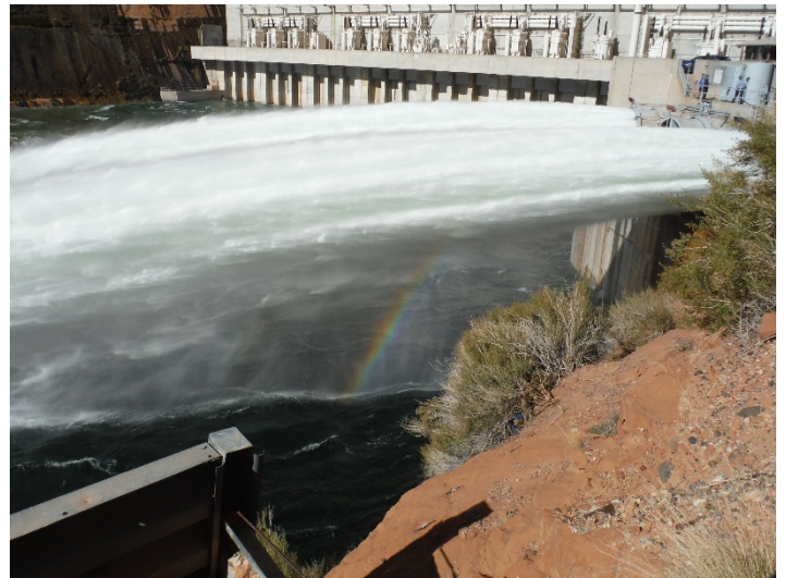
Glen Canyon Dam's Jet tubes during the high-flow experiment on November 5, 2018. (Photo credit: Todd Wojtowicz, USGS)
