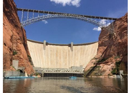
Glen Canyon Dam. (Photo Credit: Todd Wojtowicz, USGS)
