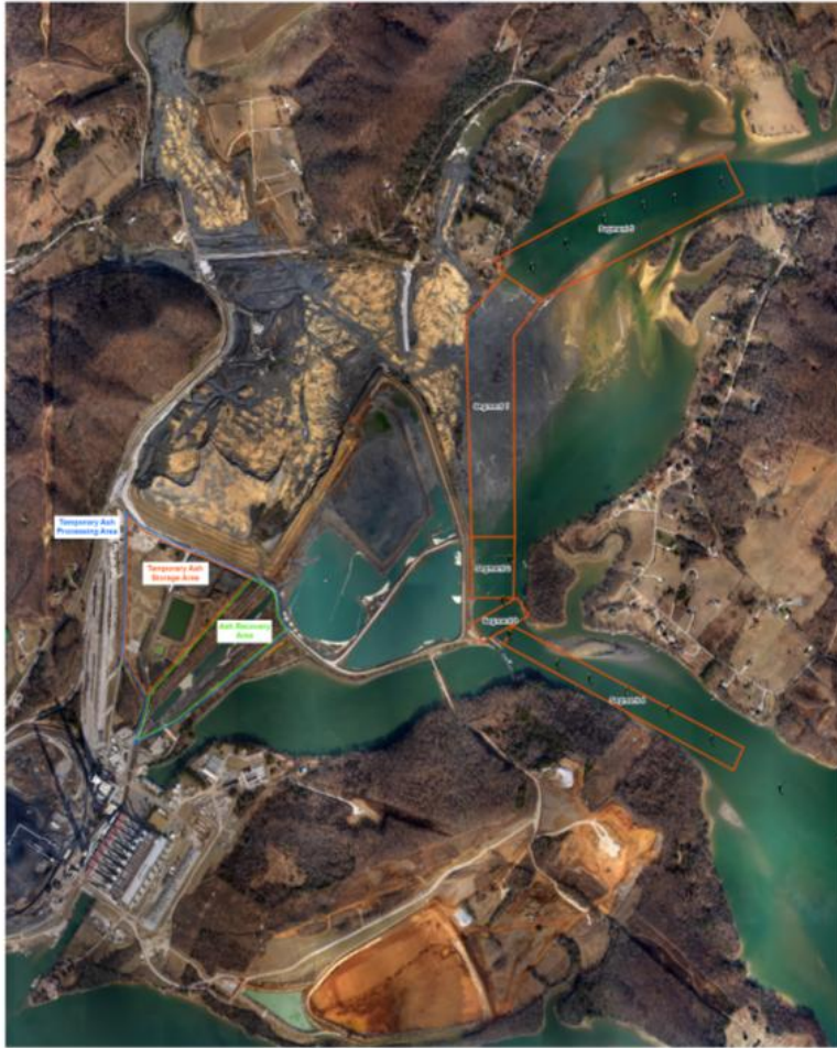
Kingston Fossil Plant Ash Recovery Project
