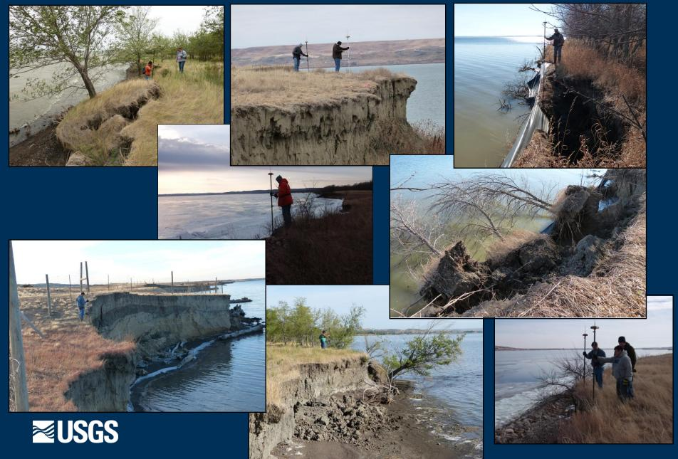
Results from the quarterly RTK monitoring were severe in many areas during the nine months from Nov., 2011 to Aug., 2012. Loss of bank ranged from zero to over 14 feet in the seven-mile study area.
