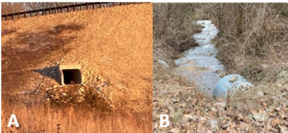
Figure 45. Examples of culverts, which can be many shapes and sizes and found in a variety of locations. Example A is a very large box culvert running underneath an interstate. Example B shows a much smaller culvert running under a two-lane residential road. (Photo credit: Christy-Ann Archuleta).
