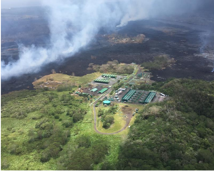
The 2018 Kīlauea Lower East Rift Zone eruption (HI) of covered 3 wells in Puna Geothermal Venture (PGV) power plant
