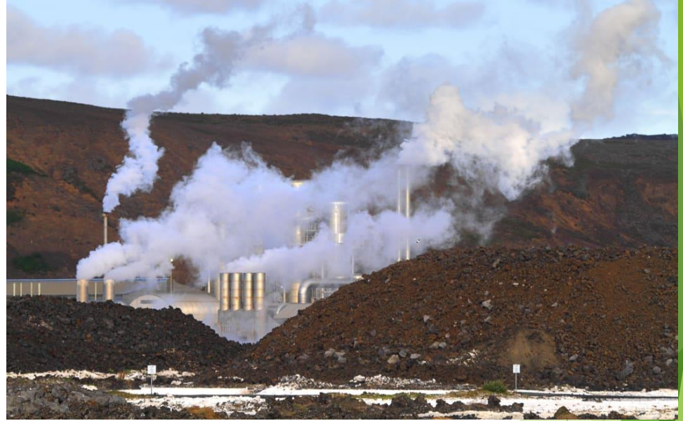
At the Svartsengi power plant in Iceland, embankments have been built and reinforced in recent years
