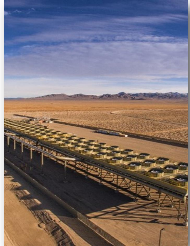
36-MW Don A. Campbell Geothermal Power Plant (Ormat), a hidden system discovered during mineral exploration drilling
